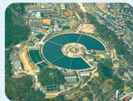
Uegahara purification plant (Nishinomiya City) (Filtration capacity: 70,000 m 3 /day)
